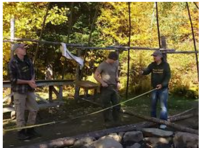
Measuring the tripod legs before tying them.
