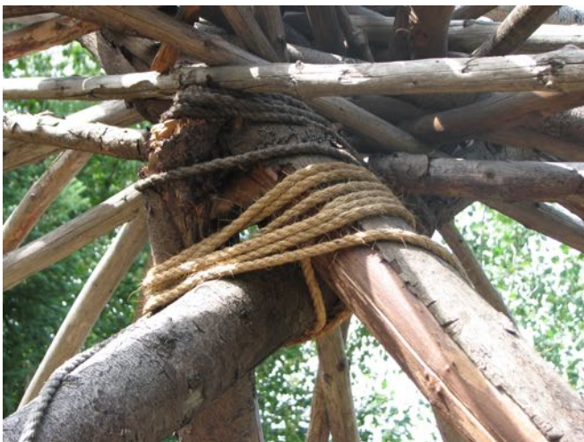
The broken tripod pole and backup rope lashing.
